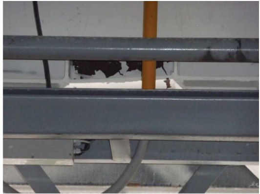
(b) Flaked paint on EBF active link with residual deformation
