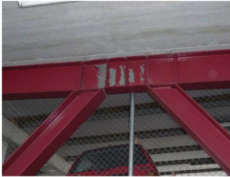
(a) Evidence of EBF link yielding
