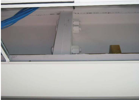
(b) Flush moment endplate splice connection
