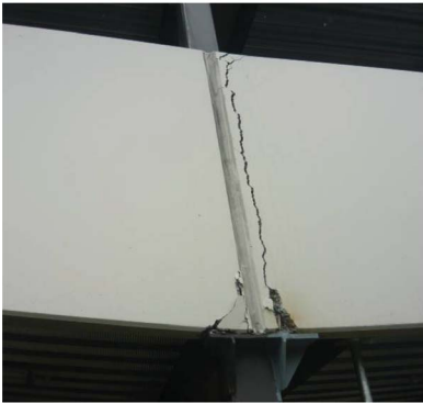
(b) Fracture of Precast Spandrel Beams on
