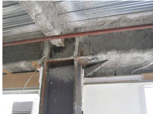
(a) Typical beam to column connection with fire protection partially removed for inspection
