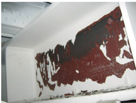
(c) paint flaking of EBF link in the ceiling space
