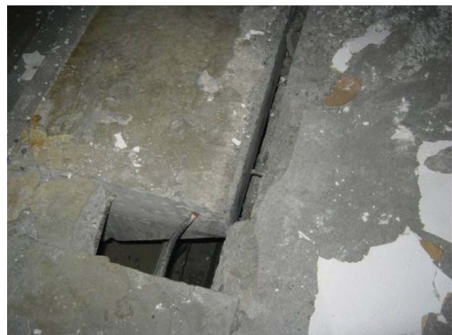
(b) Gap opening in stair at landing due to lateral movement (stairs had independent structural support).
