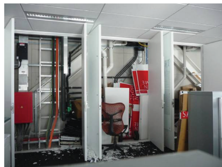
(d) global view of EBF braces obstructed by various utility runs
