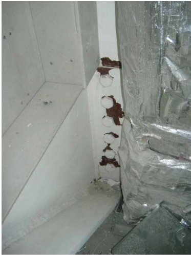
(a) Brace/beam/column connection showing out-of-plane yielding in endplate but no inelastic demand in gusset plate
