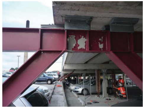
(d) Active link at top storey supporting partially completed ramp to future new level
