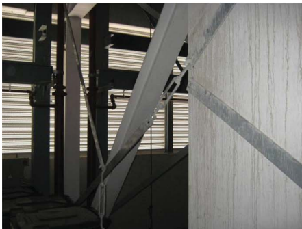
(c) Multi-story mechanical garage stacker failed braces
