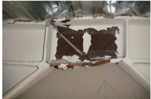
(d) Fractured EBF active link in top level of EBF system in front face of atrium
