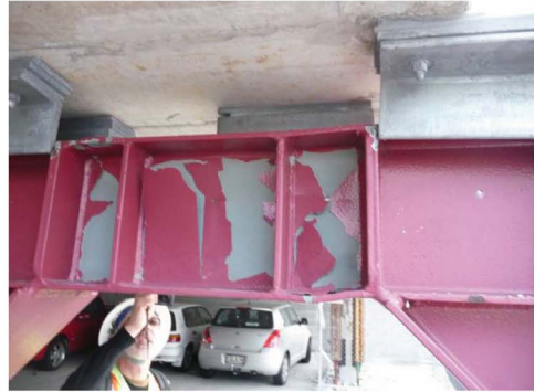
(b) One of the two active links with fractures
