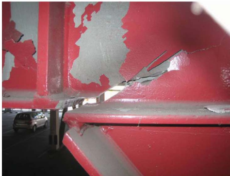
(c) Close-up view of most severely fractured active link
